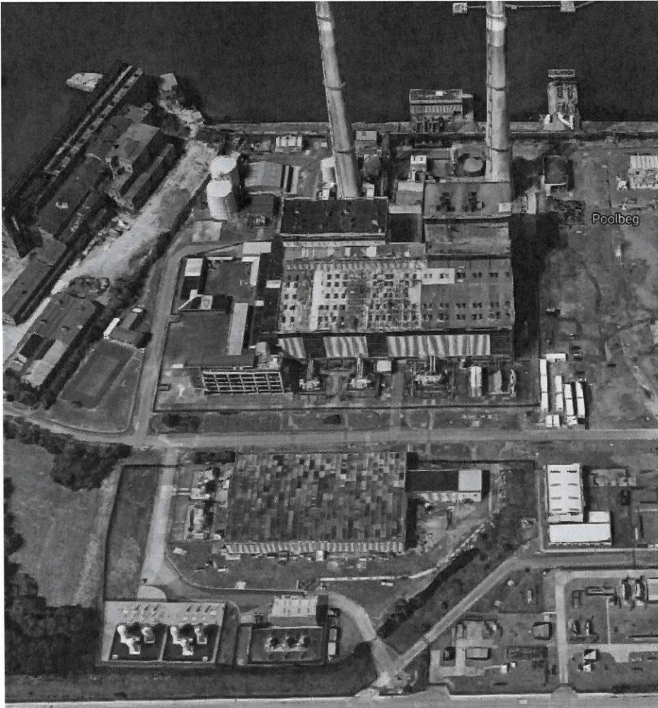
Figure 4: Image (source Google Maps) of Poolbeg (Shellybanks) substation, and a double set of Shunt Reactor units in bottom left of image
